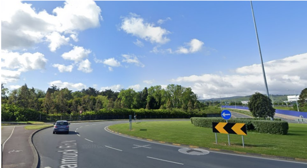
Fig. 9 Glenamuck Road North bridge meets the roundabout (Eye 2 position)
