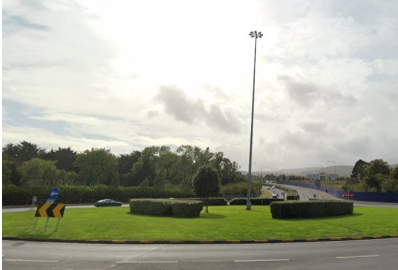
Fig. 24 Existing public lighting on the roundabout adjoining the site
